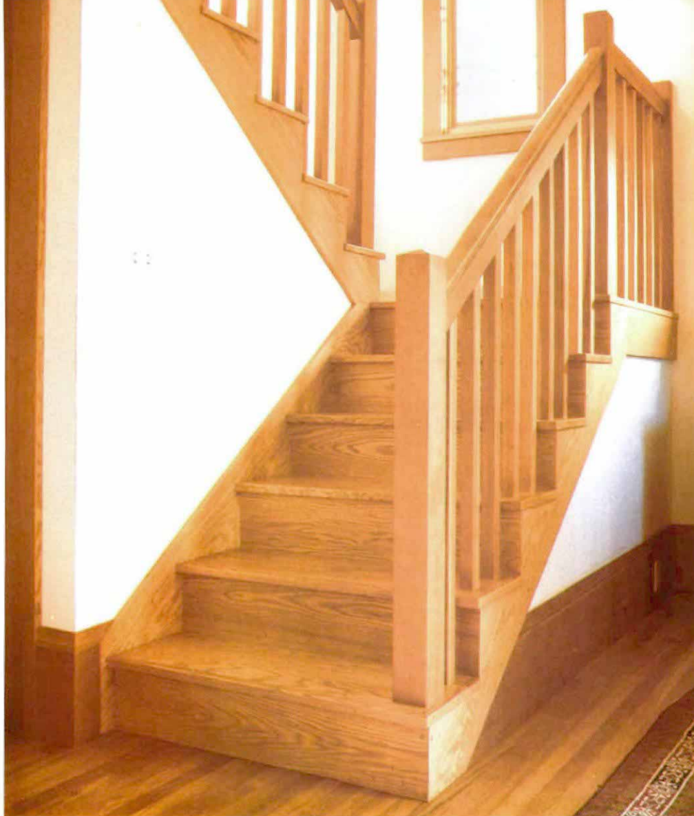
Rising from what once was a bedroom, this new stair leads to a second-story addition on a turn-of-the-century Arts and Crafts home. Builder Alexander Brennen built the stair on site, using Douglas fir newel posts, oak treads and risers to match the flooring; railings and balusters to correspond with the original trim elements.
